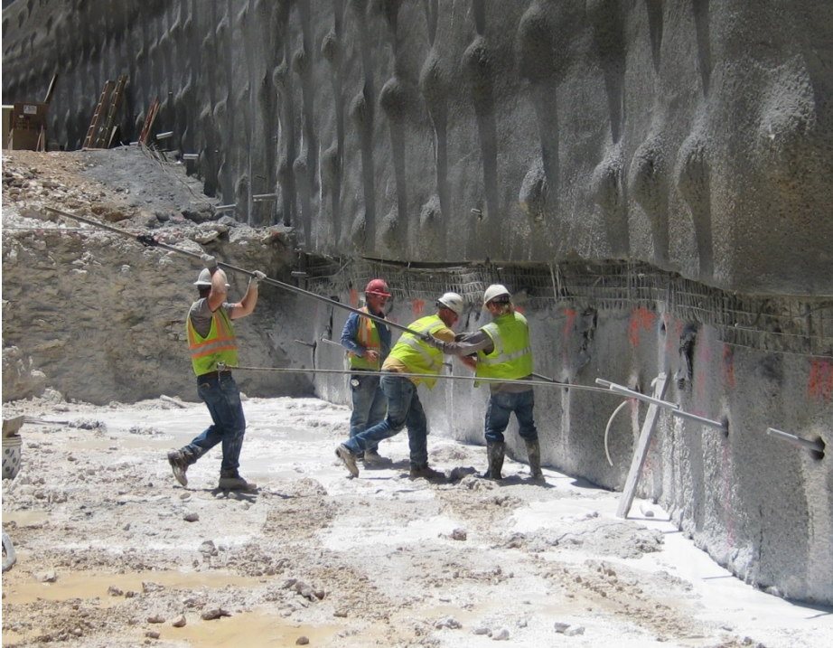
Figure 3.16: Photo. Solid nail tendon installation. Photograph courtesy of Schnabel Engineering.
