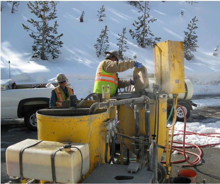
Figure 3.4: Photo. Typical grout plant setup. Photograph courtesy of Barry Siel, FHWA.
