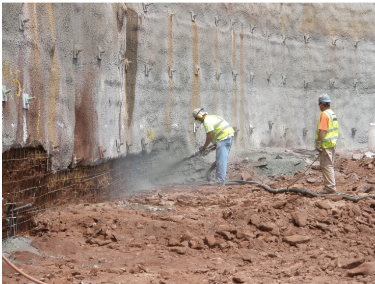
Figure 3.17: Photo. Initial shotcrete application. Photograph courtesy of Moretrench American Corporation.
