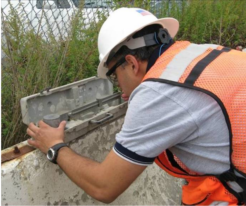
Figure 3.5: Photo. Baroid mud balance to measure specific gravity. Photograph courtesy of Schnabel Engineering.
