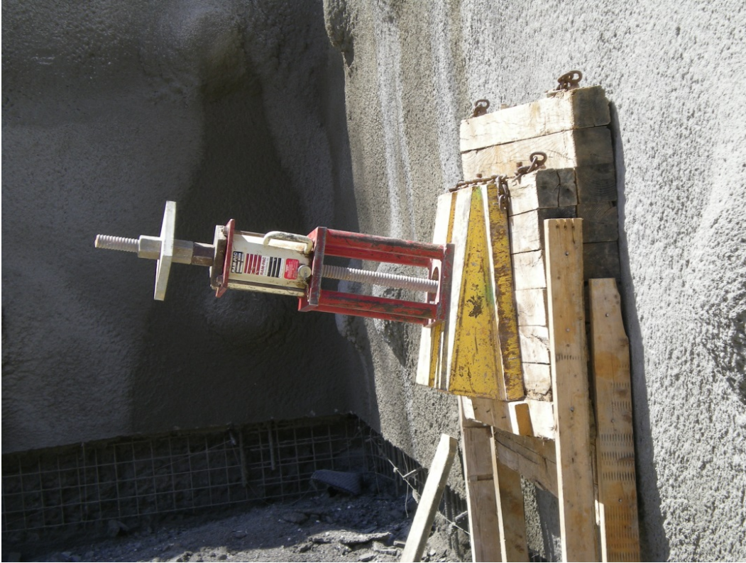
Figure 9.2: Photo. Soil nail load testing setup against shotcrete facing. Photograph courtesy of Schnabel Engineering.
