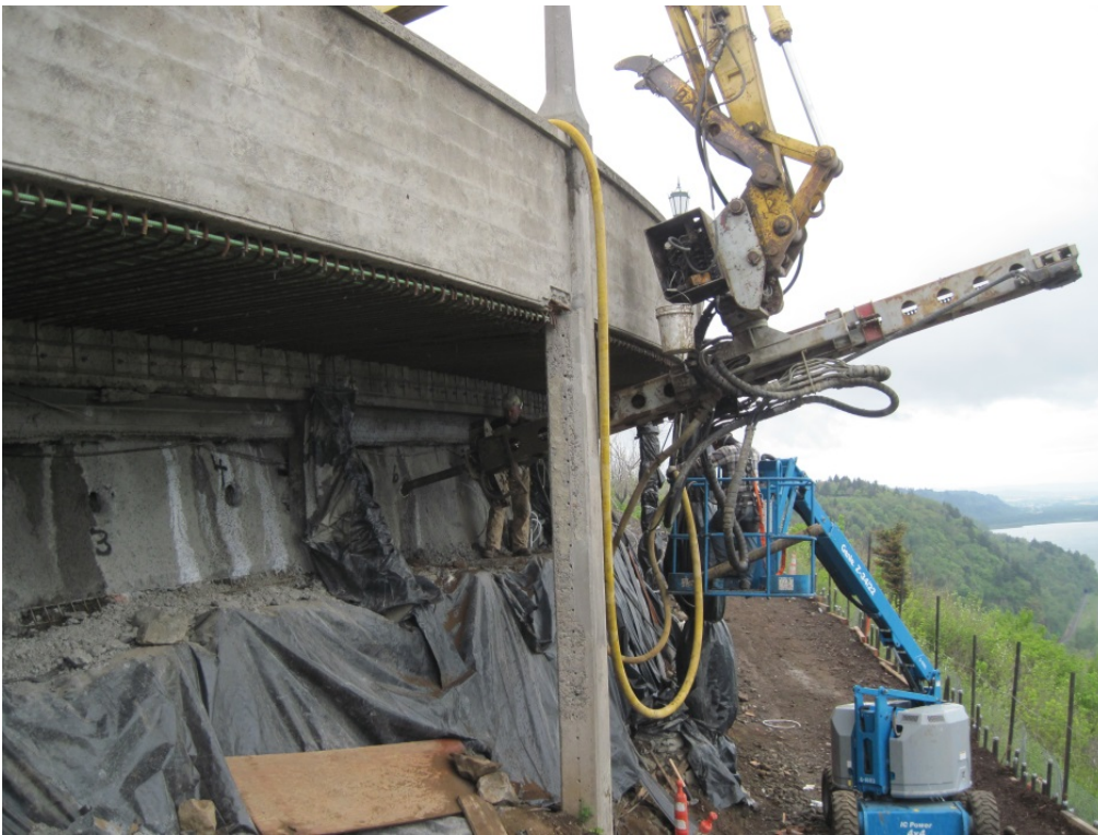
Figure 3.15: Photo. Drilling nail holes. Photograph courtesy of Barry Siel, FHWA.
