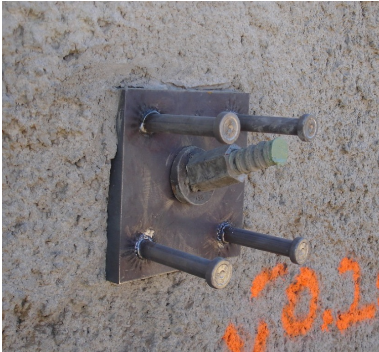
Figure 3.3: Photo. Threaded solid tendon with steel plate, washer, and nut. Note headed studs for connection to final facing. Photograph courtesy of DYWIDAG-Systems International.
