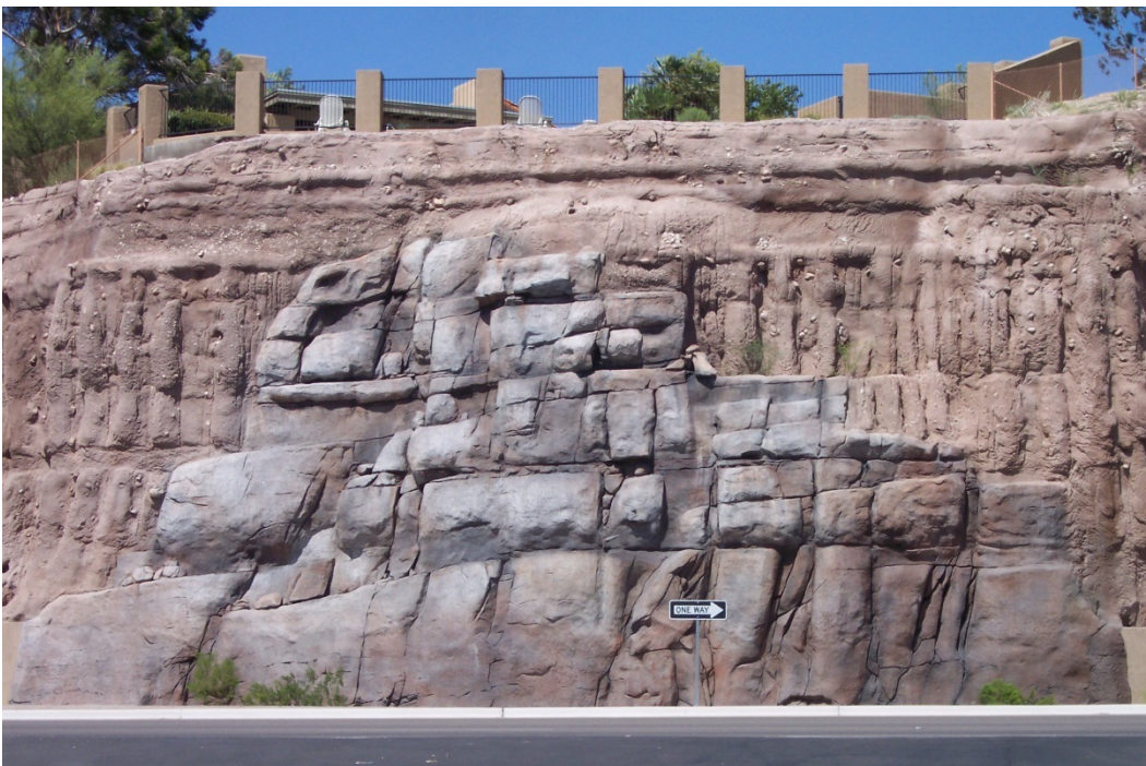
Figure 3.22: Photo. Sculpted natural rock-like wall facing. Photograph courtesy of Con-Tech Systems, Ltd.
